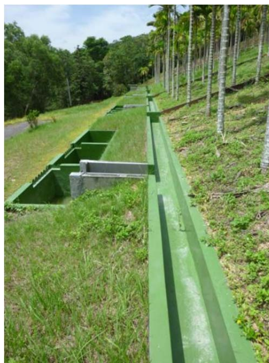
B. Flow measurement weir was set up at this site.
